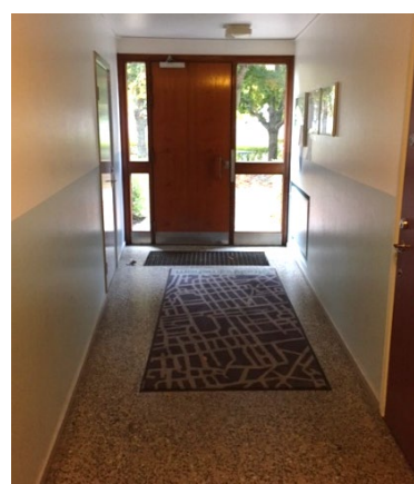
A communal hallway where service boxes will be installed
