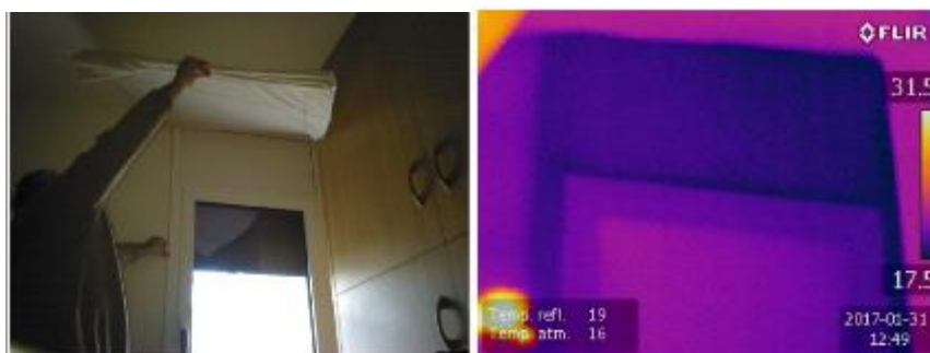
Figure 77 Thermal images after the implementation of M1.1.10.1 in Canyelles
