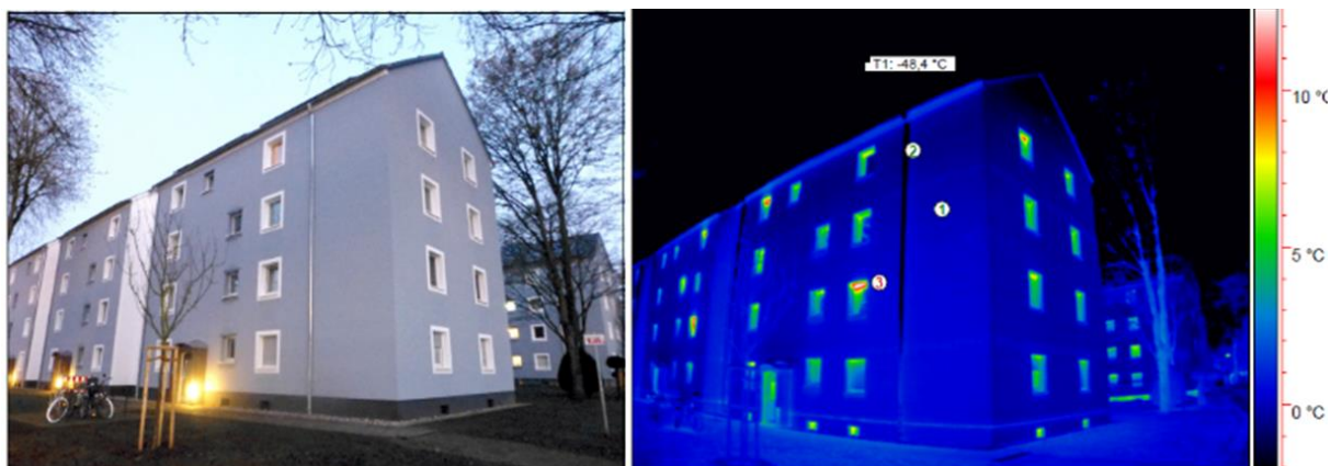
Figure 54 Example of thermographic measurements
