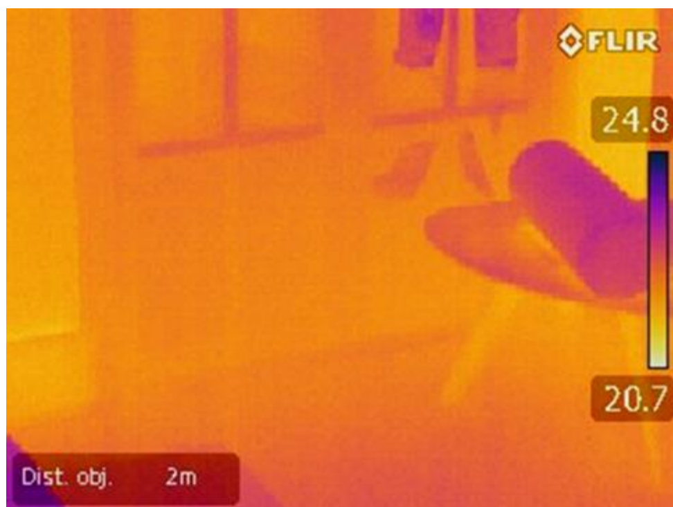
Figure 84 H10 Madison: thermal imaging after the refurbishment (installation fixed)
