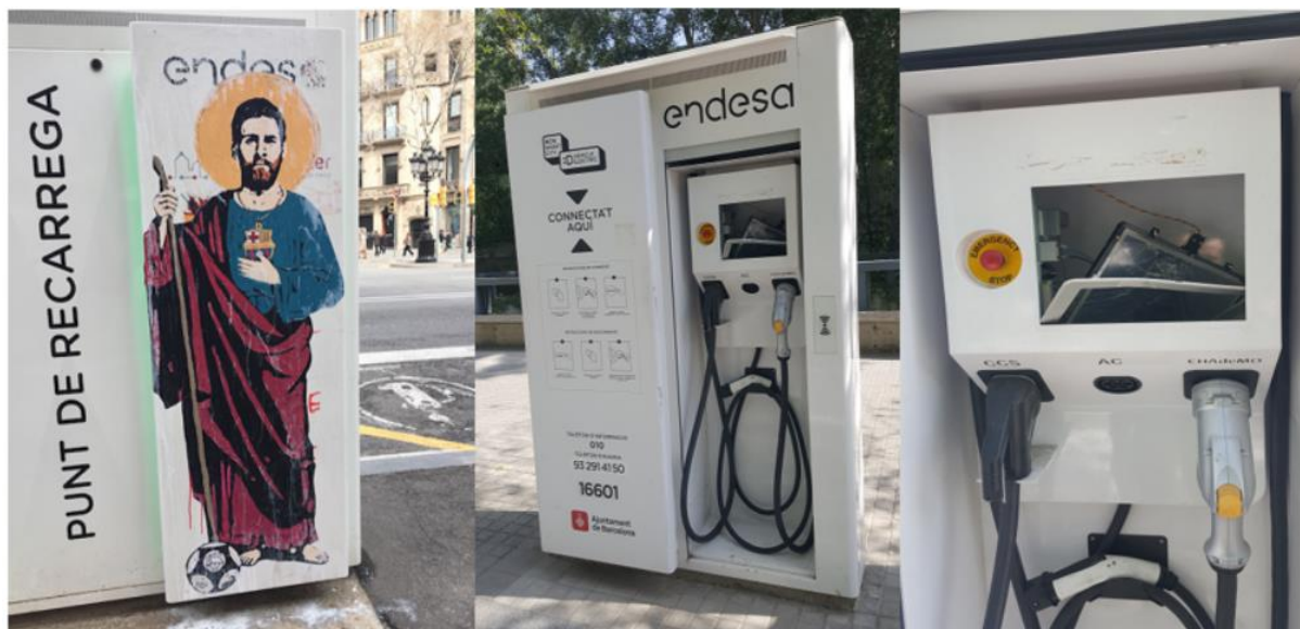
Figure 221 Examples of vandalism incidents (M11.1-M11.2)
