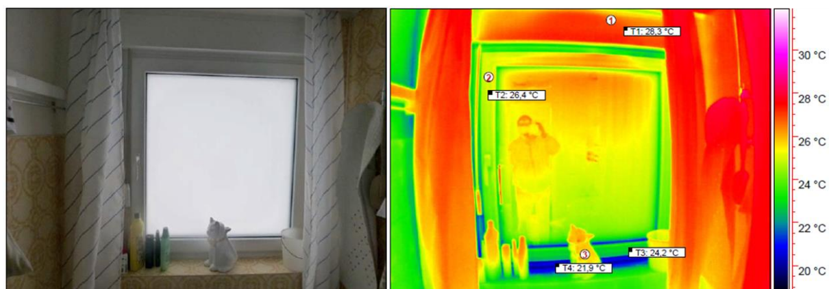
Figure 56 Example of thermographic measurements
