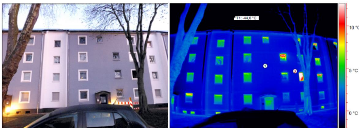
Figure 52 Example of thermographic measurements, Adam Stegerwald Straße 21
