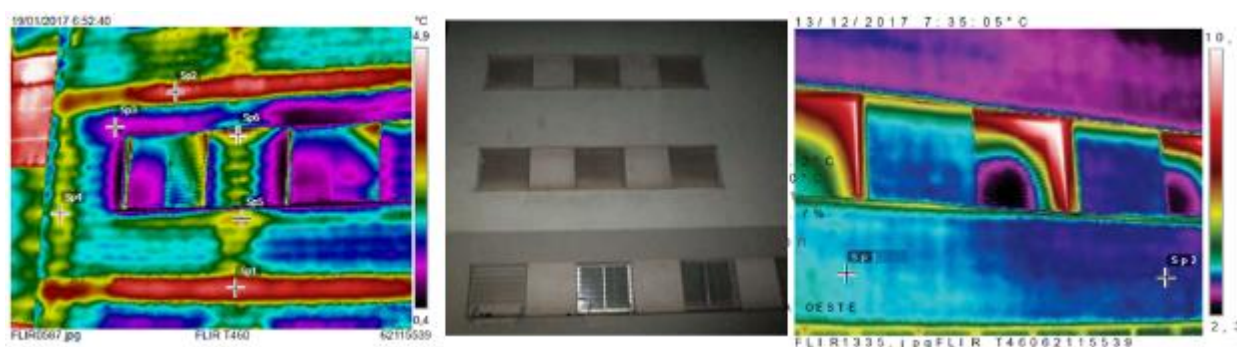
Figure 75 Thermal image of west facade before (left) and after (right) facade thermal upgrade works
