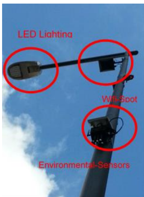
Figure 126 Details of the light pole installation in Cologne
