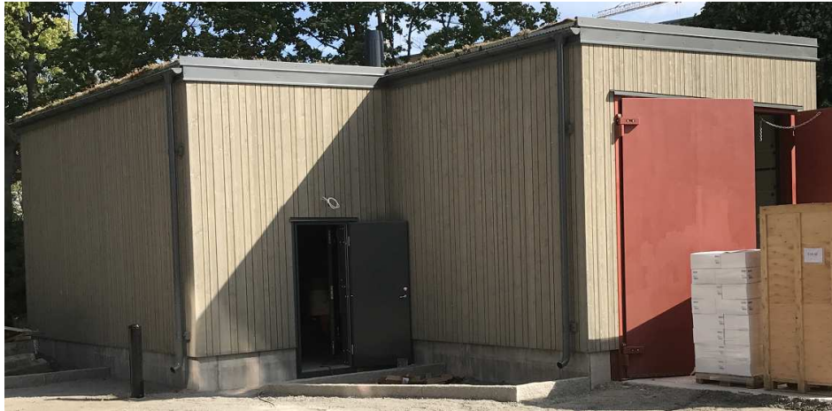
The terminal building which has the vacuum technology and storage of waste described above
