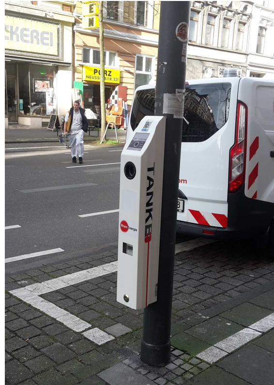
Retrofitting existing lamp posts with electric charging stations - RheinEnergie
