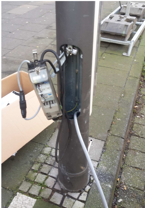
Retrofitting existing lamp posts with electric charging stations - RheinEnergie
