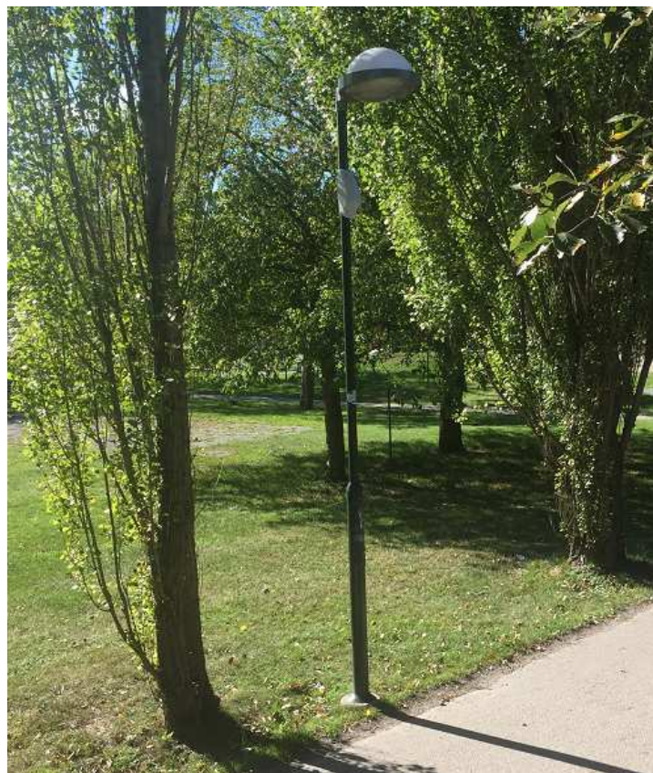
Smart Lamppost with LED and adaptive steering box on pole
