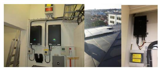
EnergyHub inverters (left), PV cells (centre), and control system (right)
