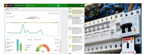
Visualization of energy consumption in Web platform (left); Sub-metering installed (right)
