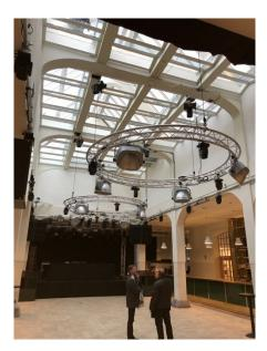
The finalised interior of the building with integrated solar panels on the outer glass roof, an insulating inner glass roof and LED lights
